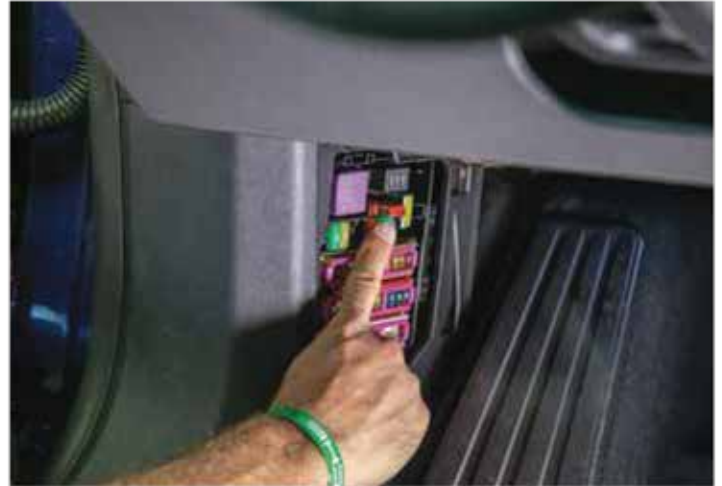
Pull out the red positive terminal. Make the 12-volt positive connection from the power source.
