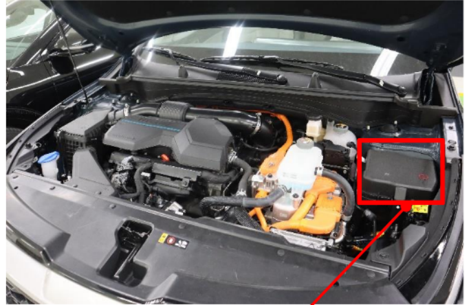
Engine room fuse box
